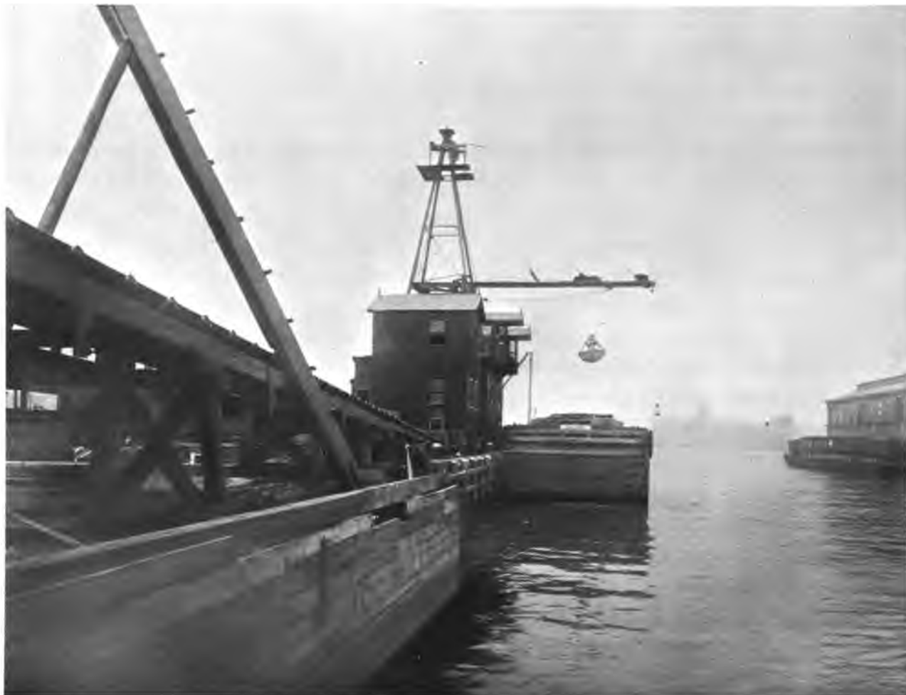
COAL UNLOADING TOWER ON WEST 58TH STREET PIER
